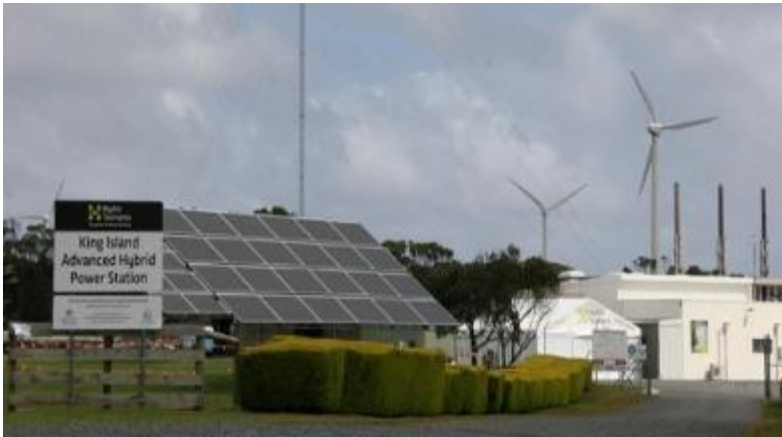
Hybrid Power Station
